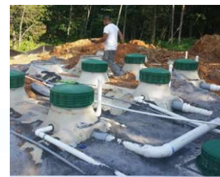
Systems may be clustered in parallel configuration for treatment of larger flows.
