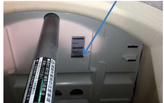
Low water line mark in sedimentation chamber
